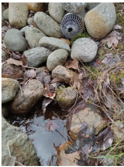
Downspout draining to pond
