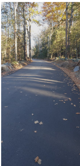
Regraded Howeville Rd., facing up from the lake. Notice slope to the right, toward culvert & away from lake. (Kathy Olson photo.)
