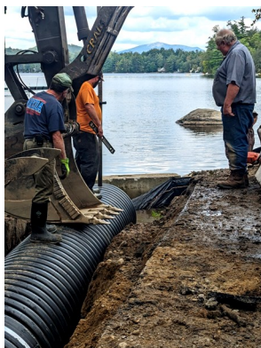
Left: Installing new culvert under Howeville Rd. (Gail Connelly photo)
