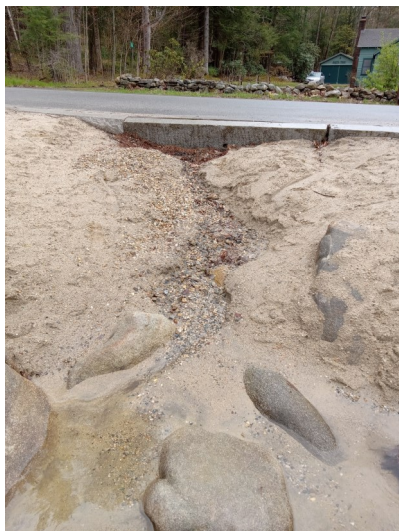
Regraded Howeville Rd., facing up from the lake. Notice slope to the right, toward culvert & away from lake. (Kathy Olson photo.)
