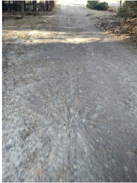
Whites Grove Rd. after regrading & new culverts. (Pat Deyo photos)
